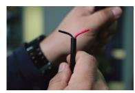
Step 8. Connect electrical. The length of wire required for final installation varies by application and is supplied by others.
