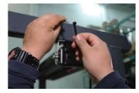
Step 6. Connect straps around brackets and tighten. Trim excess, leaving no sharp edges.
